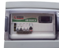
Control panel and electronic control remote
